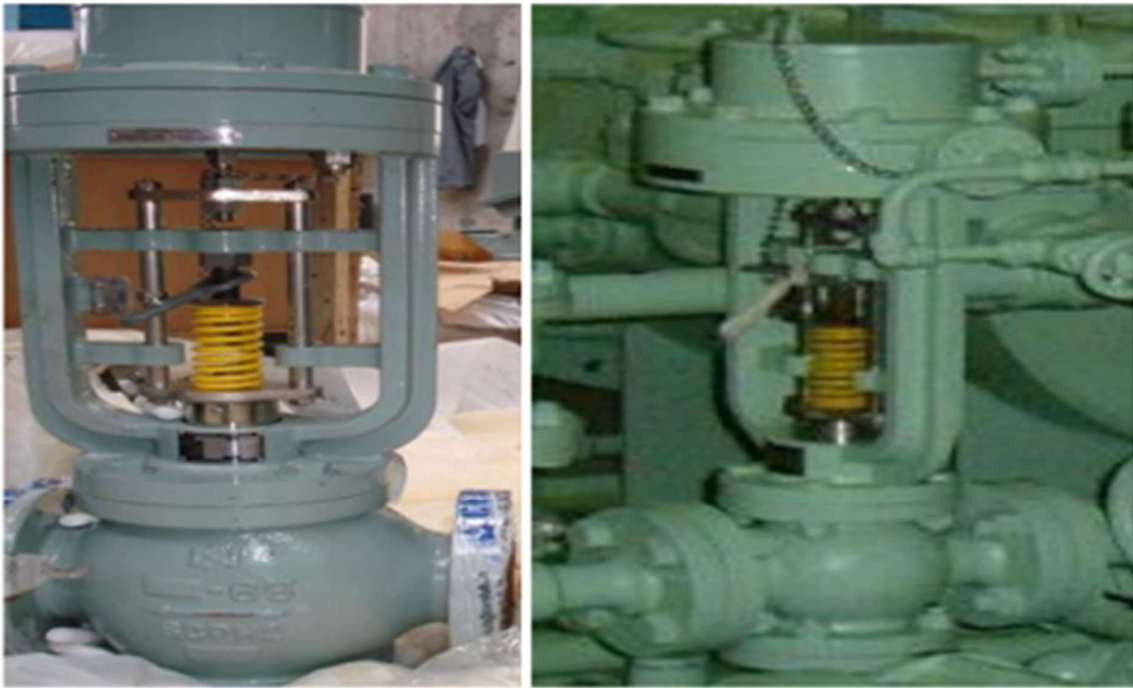
Differential Pressure Regulator (DPR) Assembly
